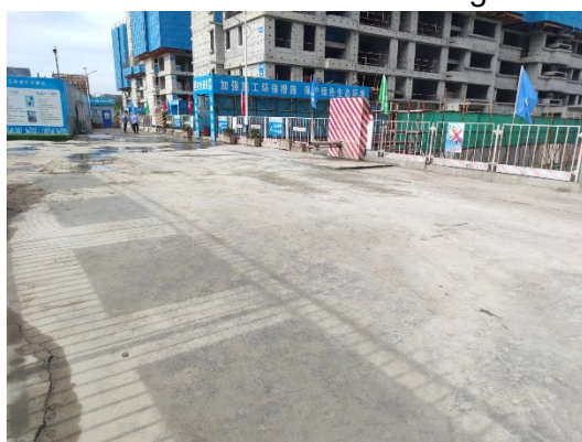
Figure 15 场地硬化
