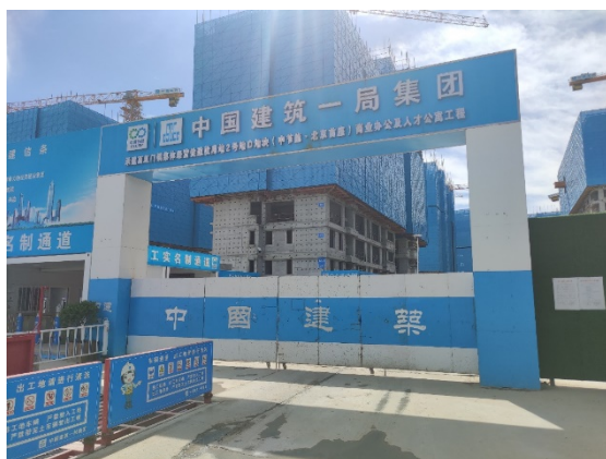
Figure 13 封闭式大门与围挡
