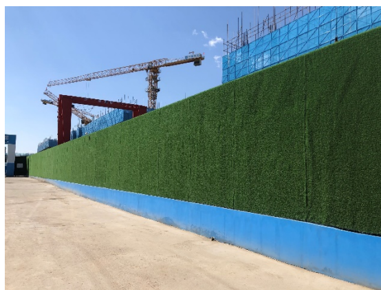
Figure 13 封闭式大门与围挡
